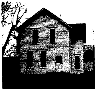
Two unit apartment house.
